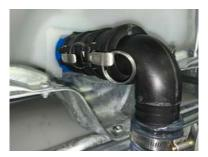
Attach the Valve Lever in position so the valve can be opened.
