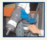
5. Secure the valve assembly with the supplied cable ties.
